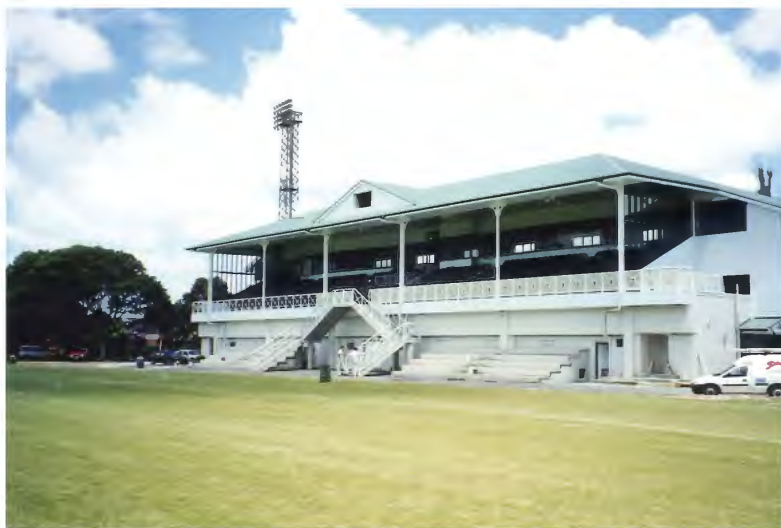
Figure 6: The new Hutt Recreation Ground Grandstand. Photo probably taken before the official opening on 12 December 1999. (Hutt City Archives, Parks and Gardens file PL12-3-HR-1/4).
