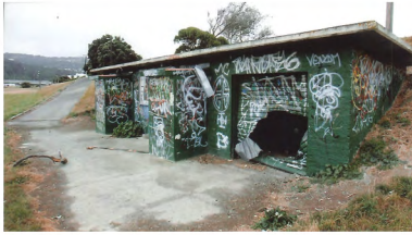
Figure 7: Changing Shed, Strand Park, 2007 (H.C. Archives).
