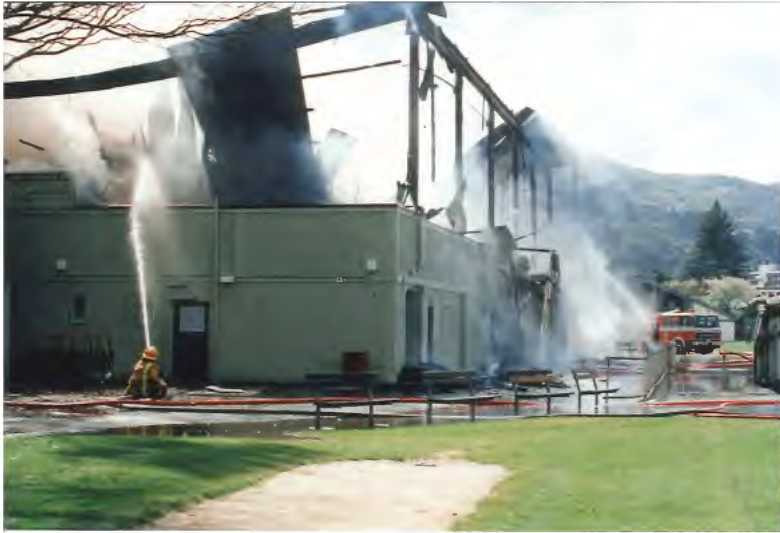
Figure 4: The smoking ruins of the old grandstand (Hutt City Council Archives, Parks and Gardens file PL12-3-HR-1/4).
