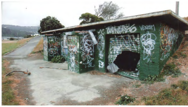
Figure 7: Changing Shed, Strand Park, 2007 (H.C. Archives).
